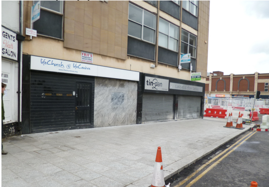
c. View east to adjacent properties
